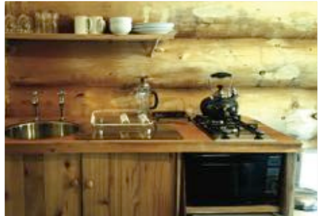
RIGHT The building includes a custom made kitchenette built from milled Western Red Cedar.
