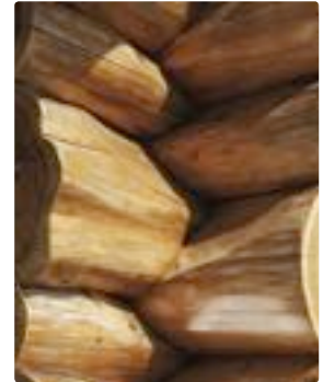
BELOW Closer look at the Scadinavian saddle notch
