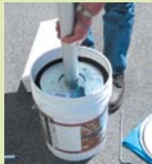
Remove the cap and cone tip from the gun barrel and push the end of the barrel onto the hole
