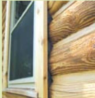
Insert Log Gap Cap™ into void between logs and frame. Leave 3/8" gap between surface of foam and edge of frame
